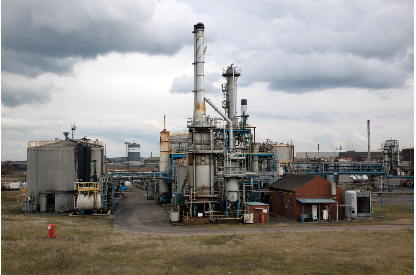
Tata Steel, Scunthorpe
