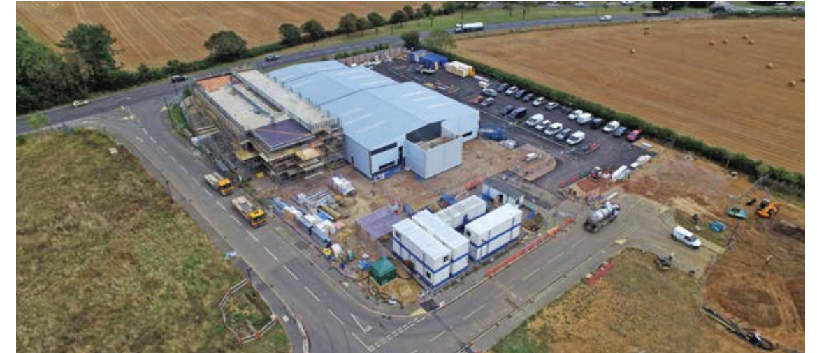
Centre of Excellence Composites Advanced Manufacturing & Marine under construction
